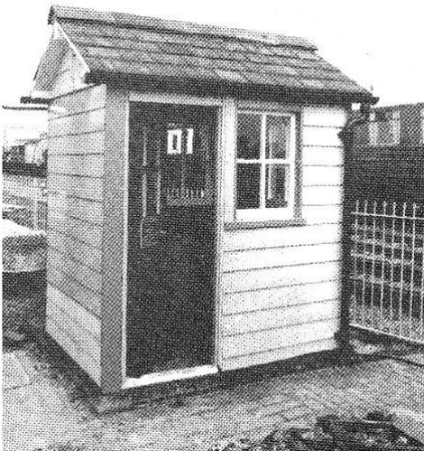
Before Holesmouth Junction Signal Box was moved to Tyseley in 1988, there had already been a small timber Signal Cabin on the site. The cabin contained a three lever Ground Frame and a telephone to communicate with the British Railways Signal Box.
