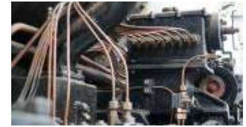
The lubricator with a small section of the complex pipework
