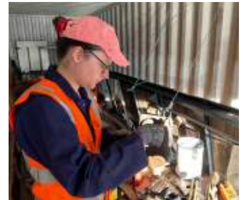
Chloe hard at work removing rust from rail connectors
