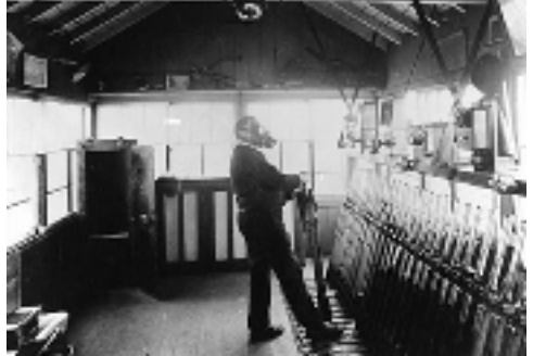
An early wartime GWR publicity photograph showing a Signalman wearing a Gas mask while undertaking his operations. An ARP Shelter can be seen in the corner of the signal box.
