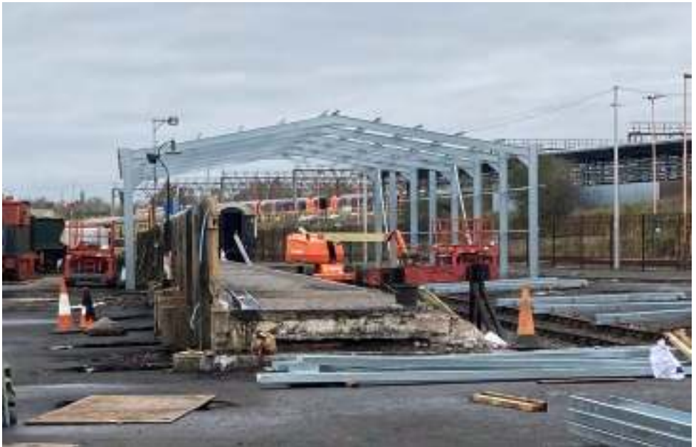
The new carriage workshop at Tyseley under construction
