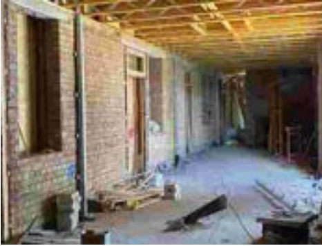
The interior of Henley station under restoration
