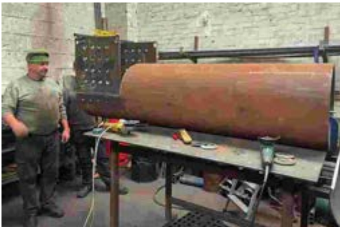
New Boiler taking shape at DLR – Pic: Andy Walton
