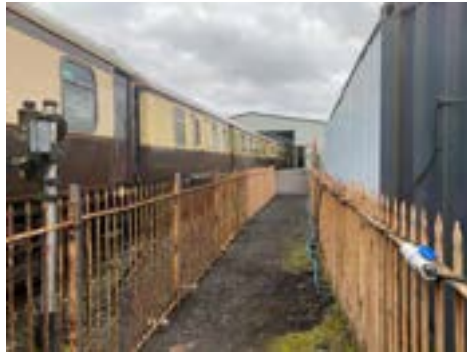
The relocated original GWR spear point railings
