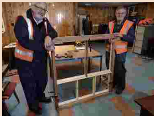
Volunteers Brian Davis and Geoff Massey progressing completion of a replacement signal box window frames in time for the depot tours.
